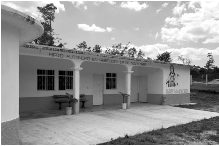
PHOTOS: FRONT PAGE: Dr. Canales, DGH's in-country project director (2nd from right), with DGH volunteers in Chiapas. ABOVE: Health clinic in Morelia.
