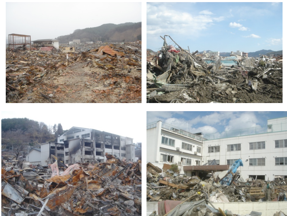
Fig 3. The center of Otsuchi-cho town two weeks after the massive Tsunami attack. The Otsuchi-cho primary school had fire (lower left) and the Otsuchi-cho hospital was destroyed as the Tsunami waves reached its second floor.
