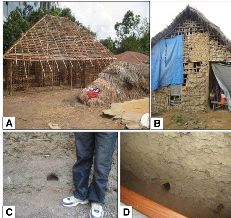
Figure 3 Typical building materials and homes made of mud and stick in rural areas of Kenema District (Panels A and B). A blue tarp provided by the United Nations High Commission for Refugees forms part of the wall in the home in Panel B. Rodent burrows can be seen in the mud foundation in the exterior (Panel C) and interior (Panel D) of houses. Photos: L. Moses.
